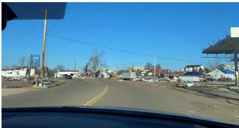
EF-3 tornado damage in Dresden, TN (Rachel Whiteman)
