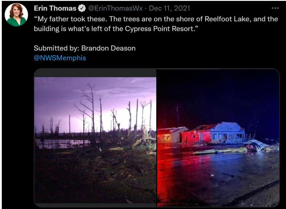
EF-4 tornado damage at Reelfoot Lake
