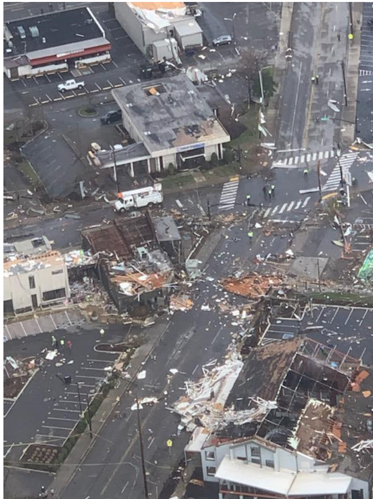
Aerial view of tornado damage in Nashville (Source: Nashville Police Department, twitter)
